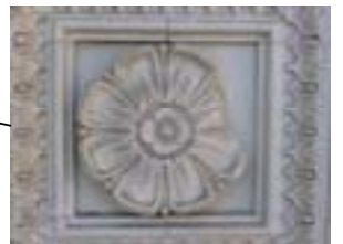
SPALLED ROSETTE COAT BROKEN EDGE
