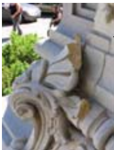
SPALLED CORNER UNIT COAT BROKEN EDGE
