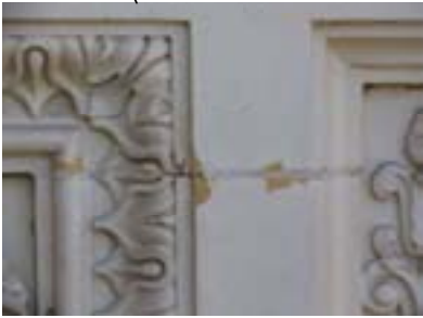
MINOR SPALLS - PATCH AND COAT
