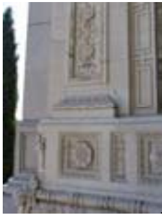
LARGE CRACK: PATCH - POSSIBLE UNIT REPLACEMENT
