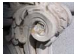
MINOR SPALL PATCH AND COAT
