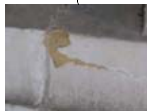
MINOR SURFACE SPALL - COAT EXPOSED BISQUE
