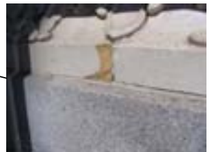
MINOR SPALL PATCH AND COAT
