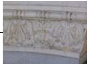
3 SURFACE SPALLS - PATCH AND COAT
