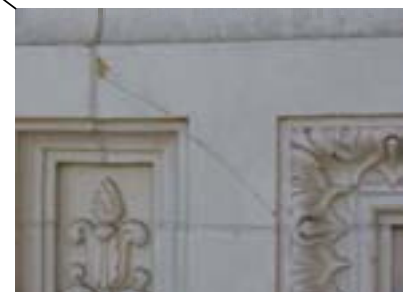
CRACK PATCH
