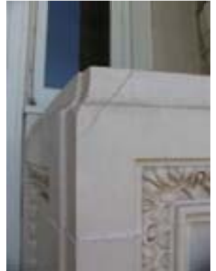
MINOR CRACK PATCH AND COAT
