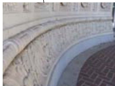
NUMEROUS MINOR SPALLS: (POSSIBLE VANDALISM) PATCH AND COAT
