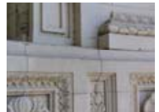
MINOR SPALLS PATCH AND COAT
