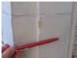
VERY MINOR SPALL - COAT EXPOSED BISQUE
