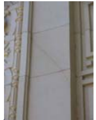
MINOR CRACK PATCH AND COAT
