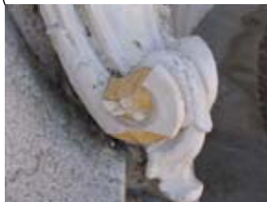
SPALLED CORNER PIECE - COAT BROKEN EDGES
