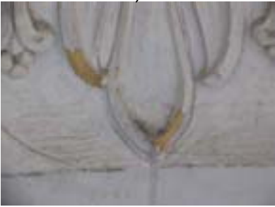
MINOR SPALLS - PATCH AND COAT
