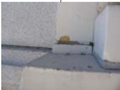
MINOR SPALL PATCH AND COAT
