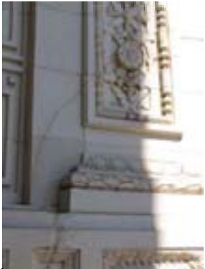
CRACK - PATCH, POSSIBLE UNIT REPLACEMENT
