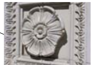
SPALLED ROSETTE - COAT BROKEN EDGE
