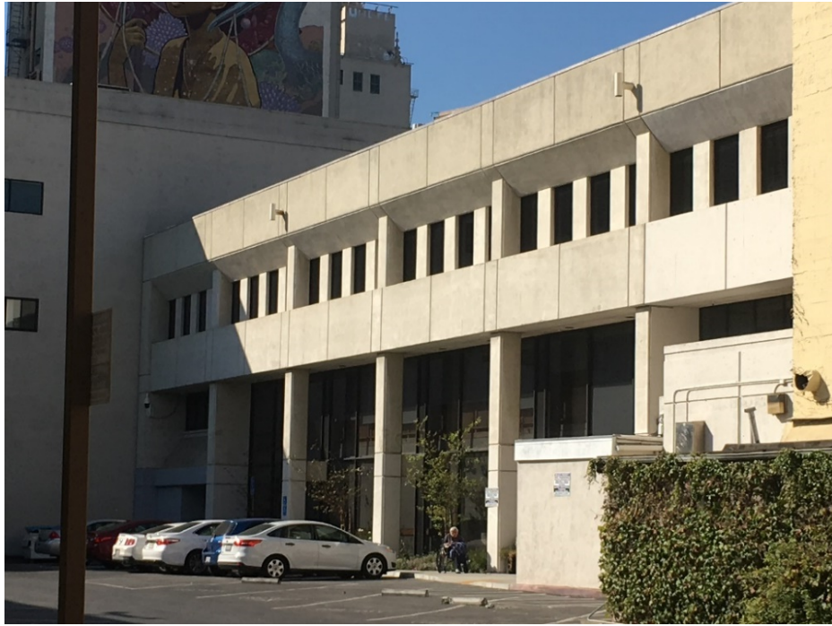
East Façade (parking lot in foreground)
