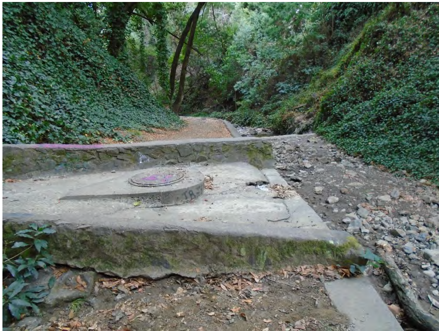
Photo 6. View facing south showing the storm water conduit and manhole. The materials on the storm water conduit have been largely replaced with, or covered by, modern concrete.
