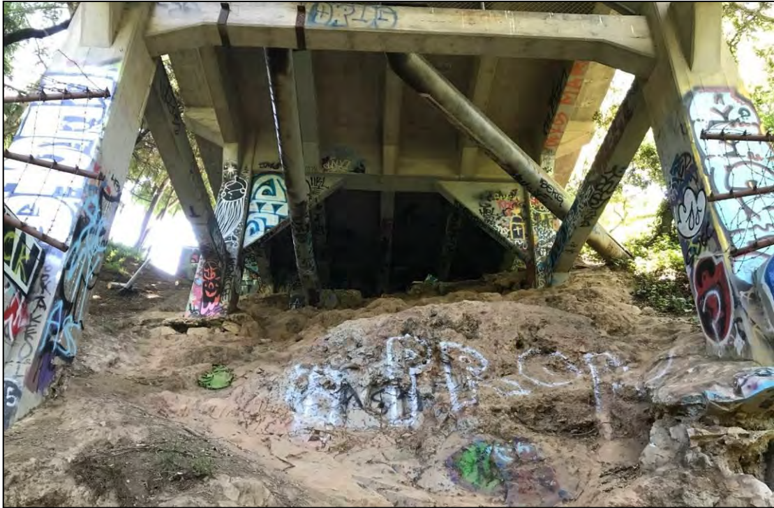
Image10: Detail view of the bridge arch from below, showing the cross bracing and the board finish, view facing east. Source: GPA, May 2017.
