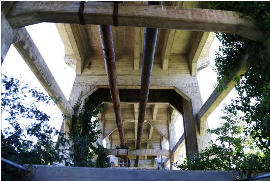
Image 12: View of the utility lines, cross bracing, and bottom of the deck, view facing northwest. Source: BCA, Inc. July 2016.
