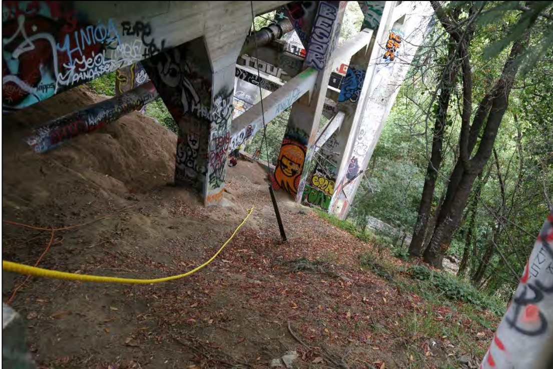
Image 12: Image showing soil erosion and footings at Bents 14 (right of frame), 15, and 16 (left of frame), view facing southwest. Source: BCA, Inc. July 2016.
