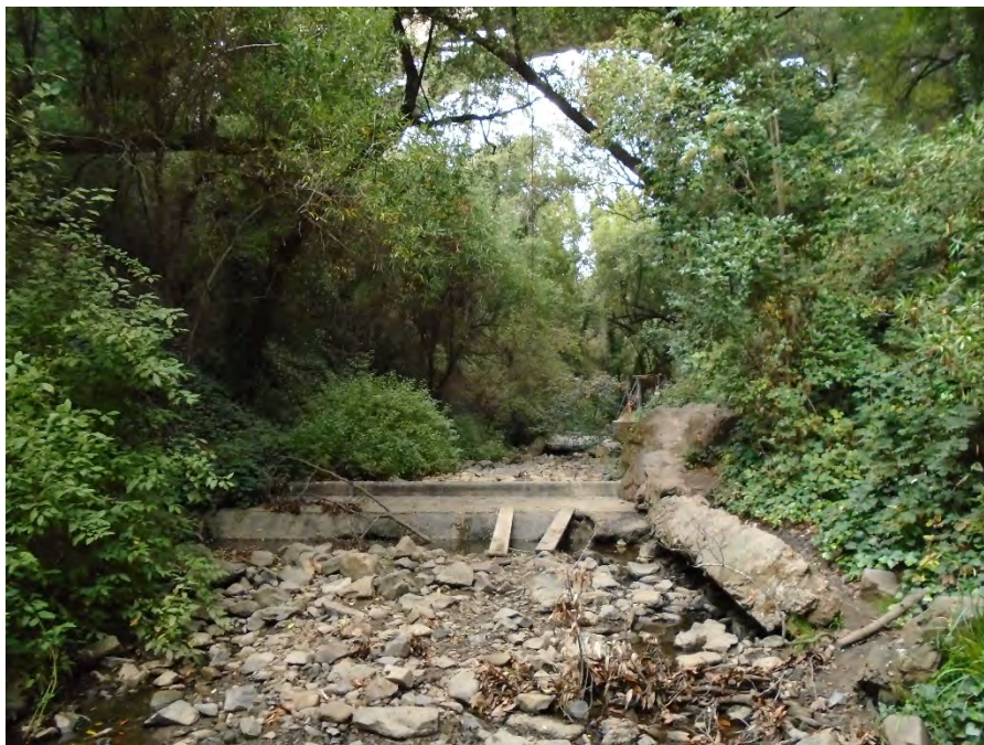
Photo 2. View facing north-northeast showing collapsed and repaired stone walls and two concrete weirs (one in foreground, one in background). The weir in the foreground has a curved dam crest and the retaining wall to the southeast of the weir has collapsed.
