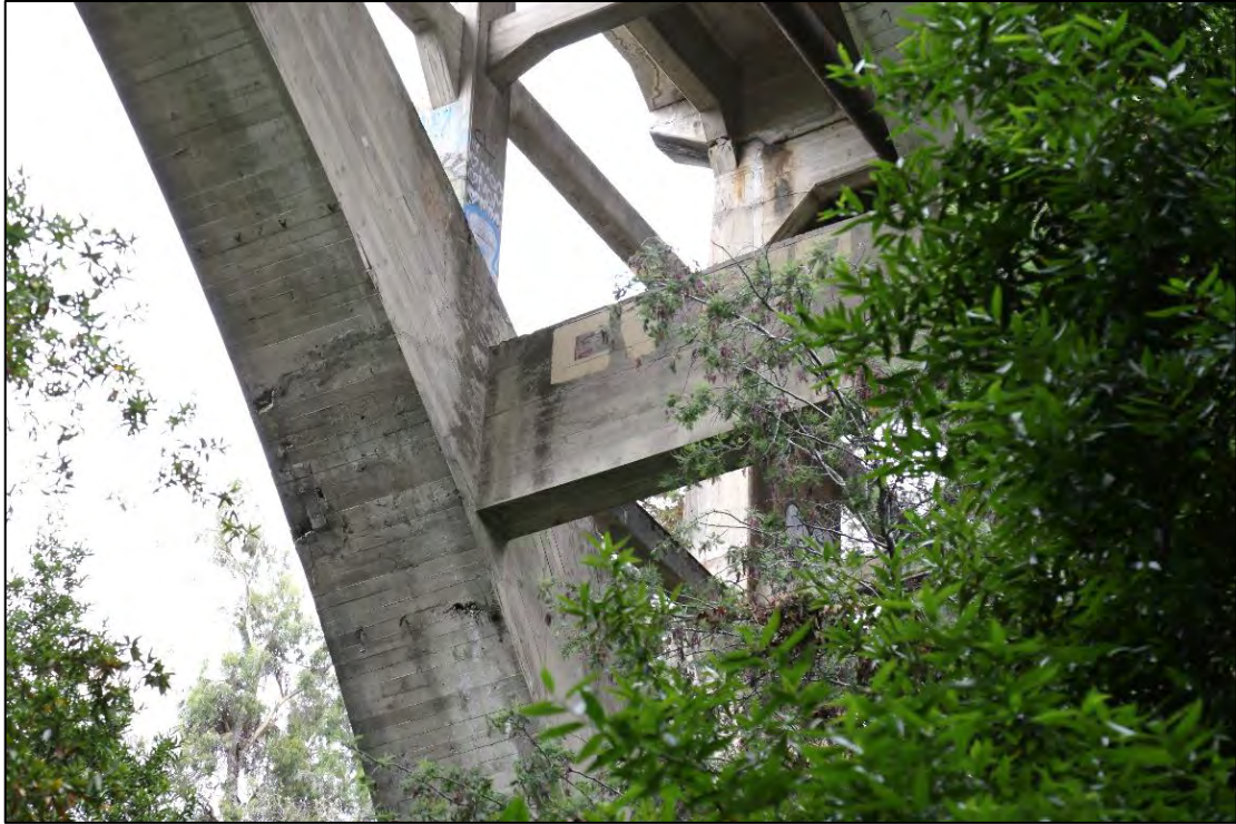
Image 10: Detail view of the bridge arch from below, showing the cross bracing and the board finish. Source: BCA, Inc., July 2016.
