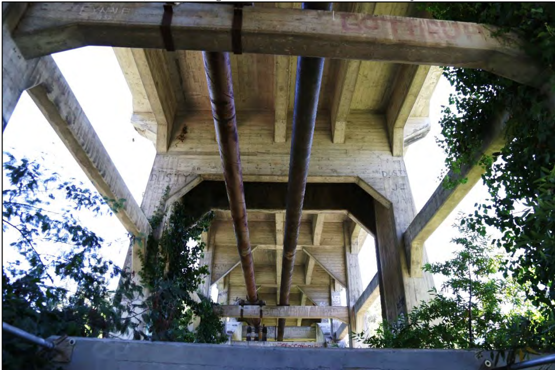
Image 13: View of the utility lines, cross bracing, and bottom of the deck, view facing northwest Source: BCA, Inc. July 2016.
