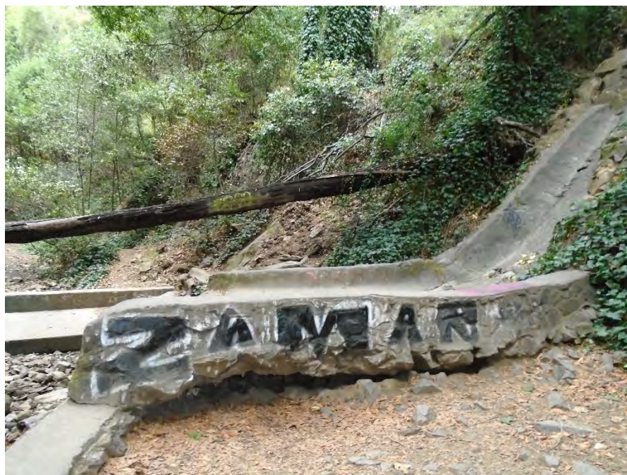
Photo 5. View facing north showing the storm water conduit. Note the scour below the retaining wall at the foreground. The weir from Photo 4 is visible in the background at the left of the frame.
