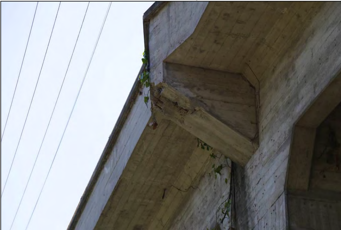
Image 13: Representative image showing typical spalling. Source: BCA, Inc. July 2016.
