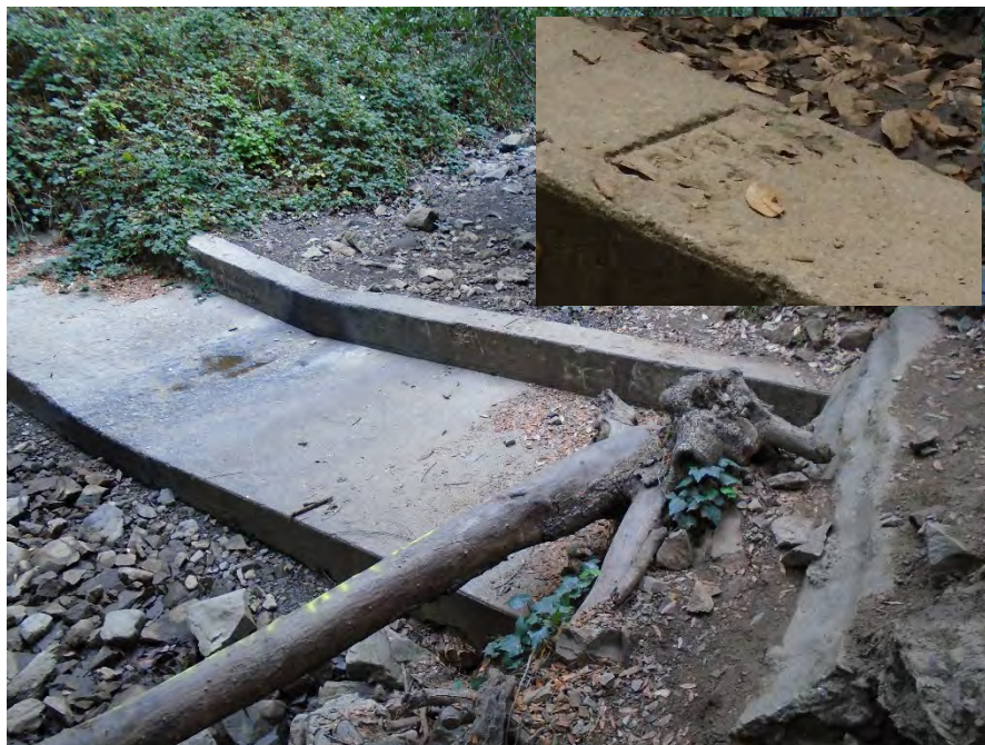
Photo 4. View facing northwest showing the northernmost weir. Note that the crest and spillway are constructed of board-formed, poured-in-place concrete. The date stamp (shown in the inset) is 1940.
