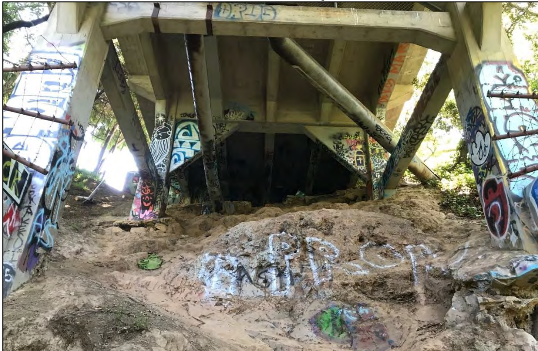
Image 11: Detail view of the bridge arch from below, showing the cross bracing and the board finish, view facing east. Source: GPA, May 2017.
