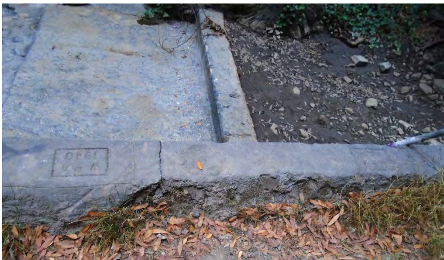
Photo 3. View facing northwest showing the weir just north of the Leimert Boulevard Bridge. The spillway of this weir has partially collapsed and has been coated with a bituminous material. The date stamp on the retaining wall just east of this weir is 1940.
