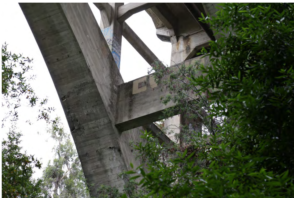
Photo 4. Detail view of the bridge arch from below, showing the cross bracing and the board finish. Source: BCA, Inc., July 2016.
