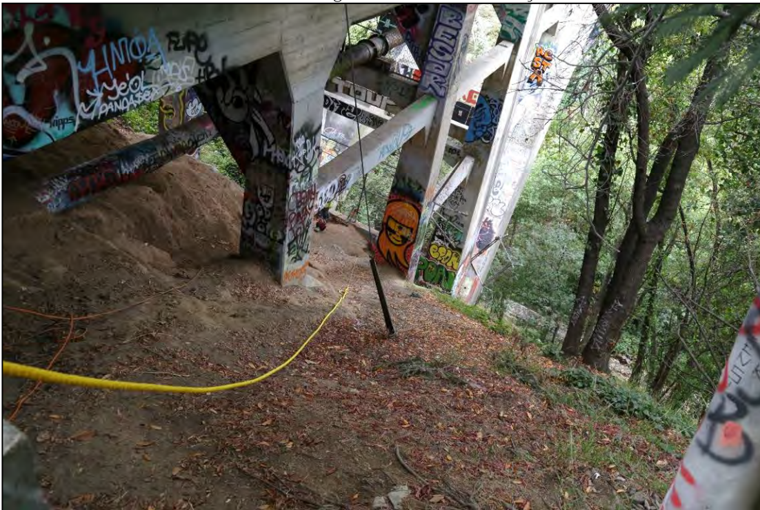
Image 11: Image showing soil erosion and footings at Bents 14 (right of frame), 15, and 16 (left of frame), view facing southwest. Source: BCA, Inc. July 2016.
