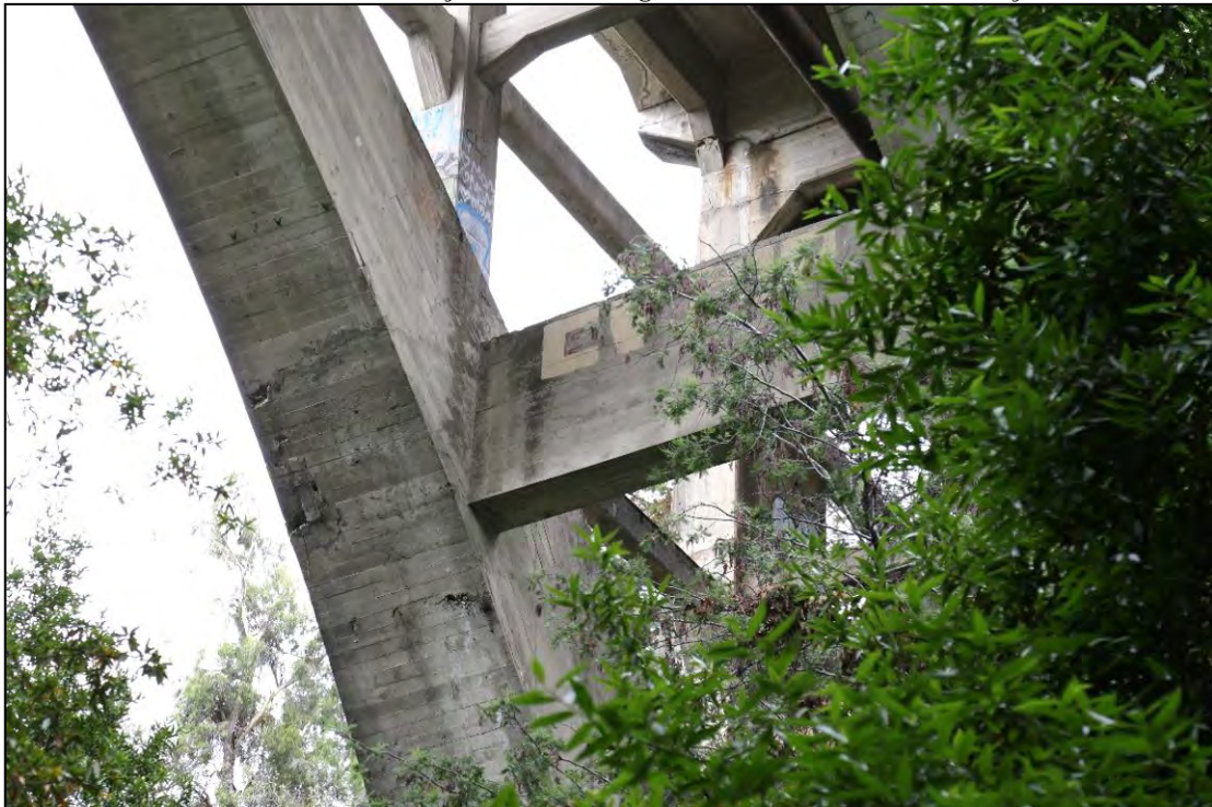
Image 9: Detail view of the bridge arch from below, showing the cross bracing, examples of spalls, and the board finish. Source: BCA, Inc., July 2016.
