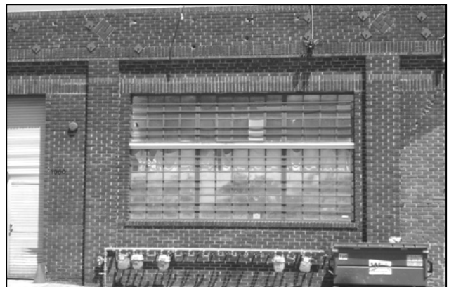
The multi-paned windows appear to be in their original metal sash design. Flat-iron bars were installed after construction of the original windows, probably for security purposes.
