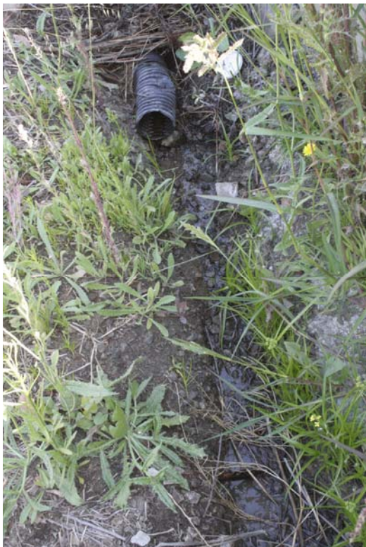
Figure 3. Corrugated drain pipe carrying subsurface flow from lots above the road
