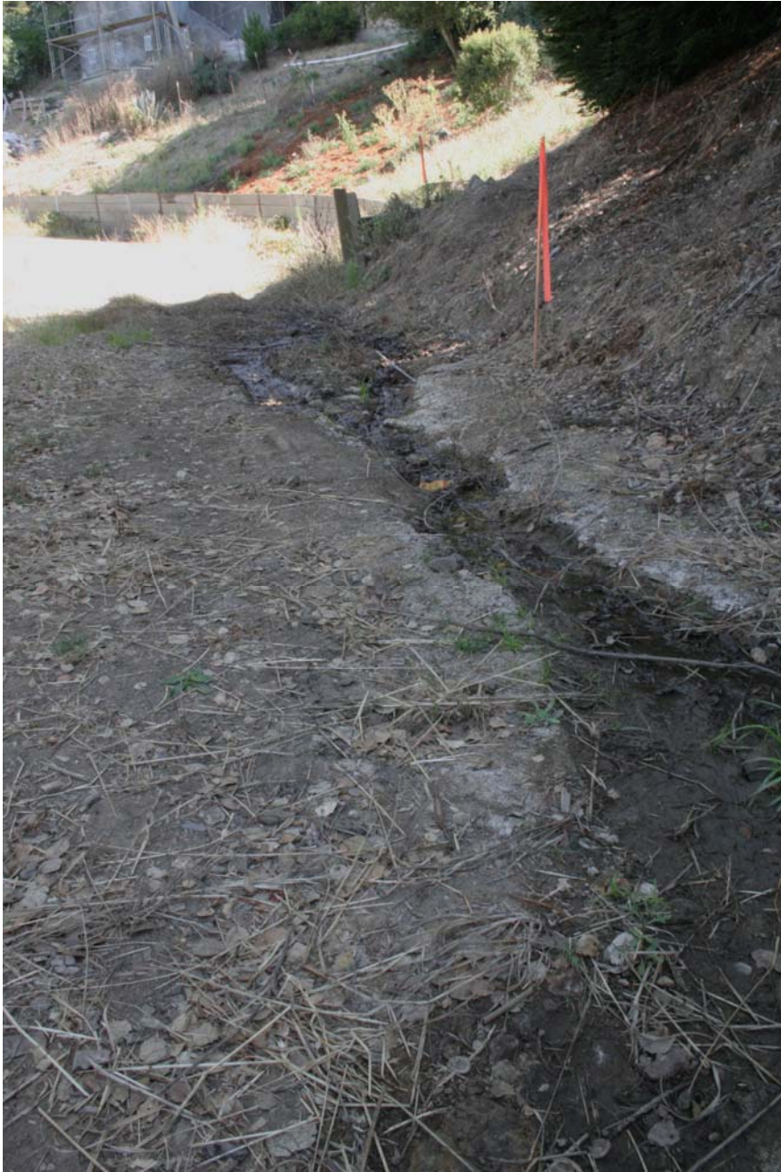
Figure 1. Water from subsurface seepage captured by the road.
