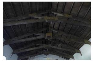
Figure 32: Scissor trusses, 2013.
