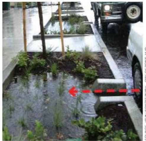
Figure 7-10 The side wings of this standard curb cut help retain the side slope grade on each side of the curb cut opening.
