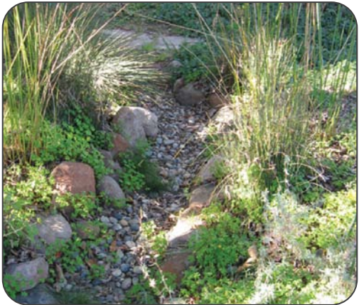
Dry creek infiltrates and conveys runoff.
