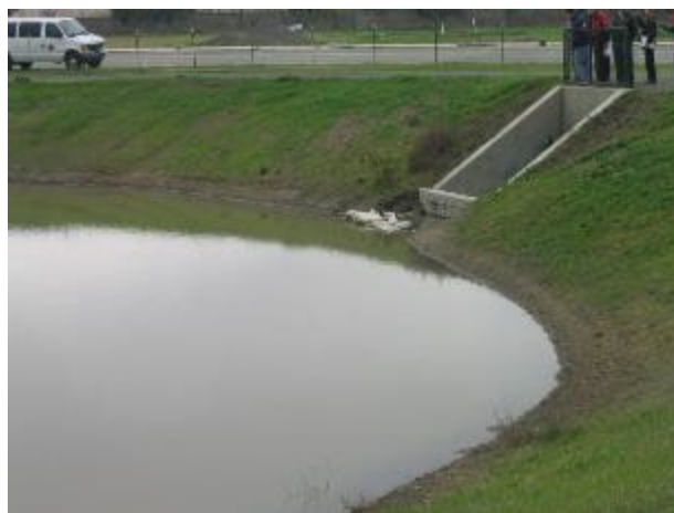
Figure 7-5 Detention pond in Pleasanton provides hydromodification management.
