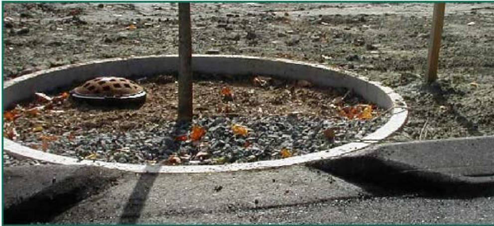
Figure 8-18 Non-proprietary Tree Well Filter with Overflow Bypass
