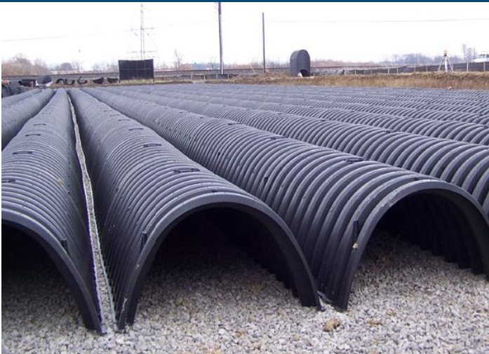
Figure 8-44 Subsurface Retention/Infiltration System Installation Under a Parking Lot
