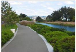
Figure 3.9.e: Asphalt is allowable if contained within flush Portland Cement headers. Provide attractive landscaping along the edges of the Bay Trail pathway wherever practicable.
