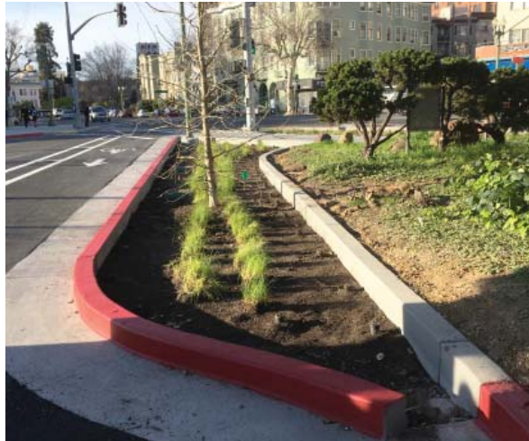
Stormwater curb extension
