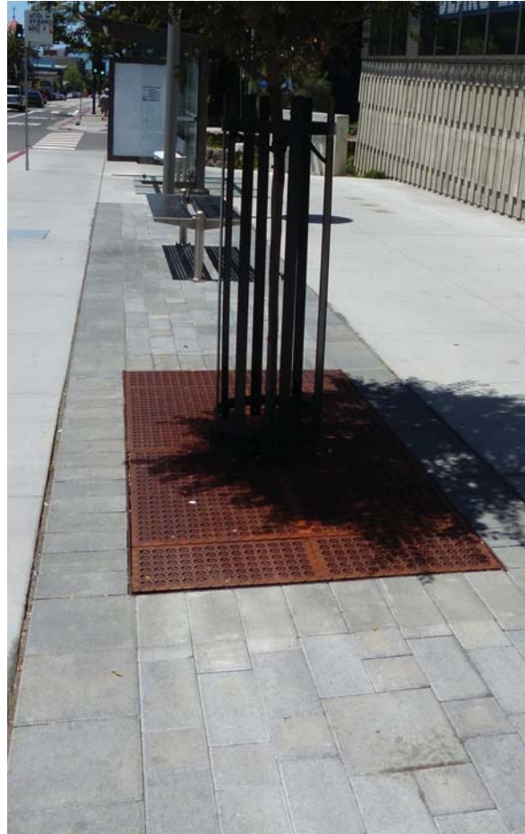
Bus stop with pervious pavers and tree well
