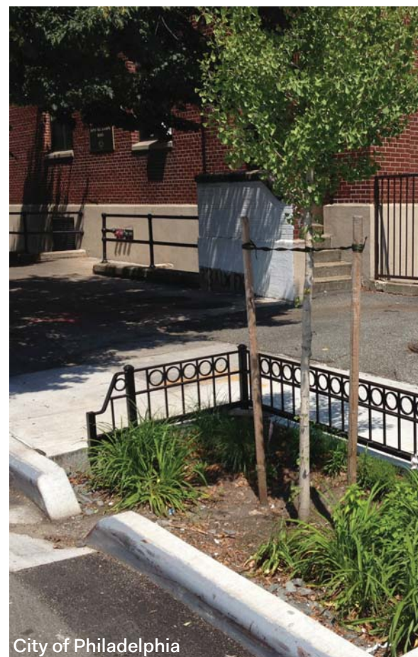
Figure 5-7. stormwater-enhanced Street Tree installation.
