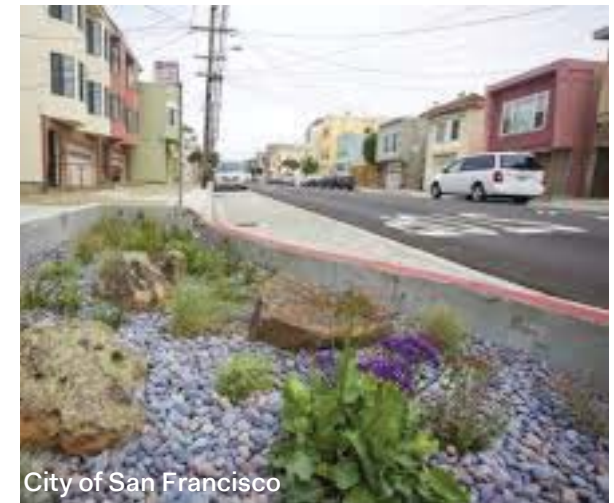
City of San Francisco Parking lane constructed of porous concrete (beyond stormwater curb extensions in foreground)
