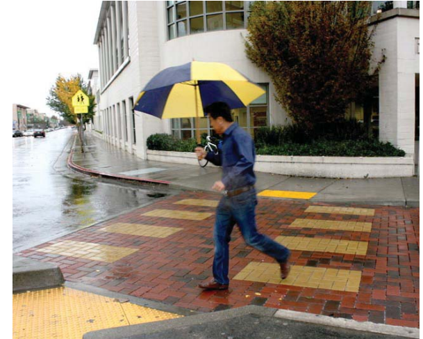
Permeable paver installation in a crosswalk
