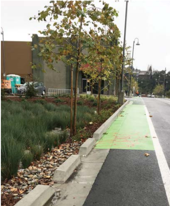
Rain garden adjacent to a bike lane
