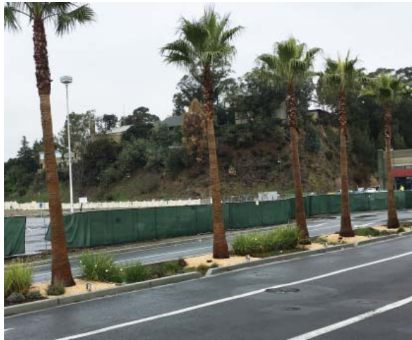
Bioretention areas and regular landscaping combined in a single median
