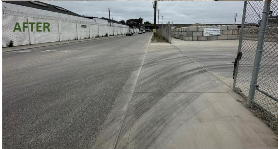
Sediment cleared, and sediment tracking controls installed at truck exit
