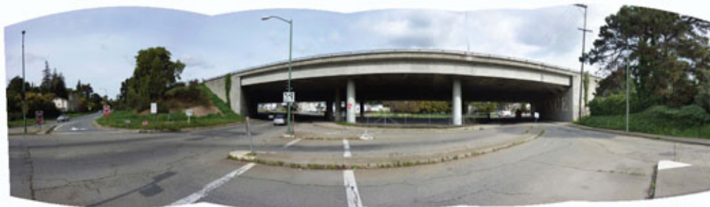
View of underpass looking north
