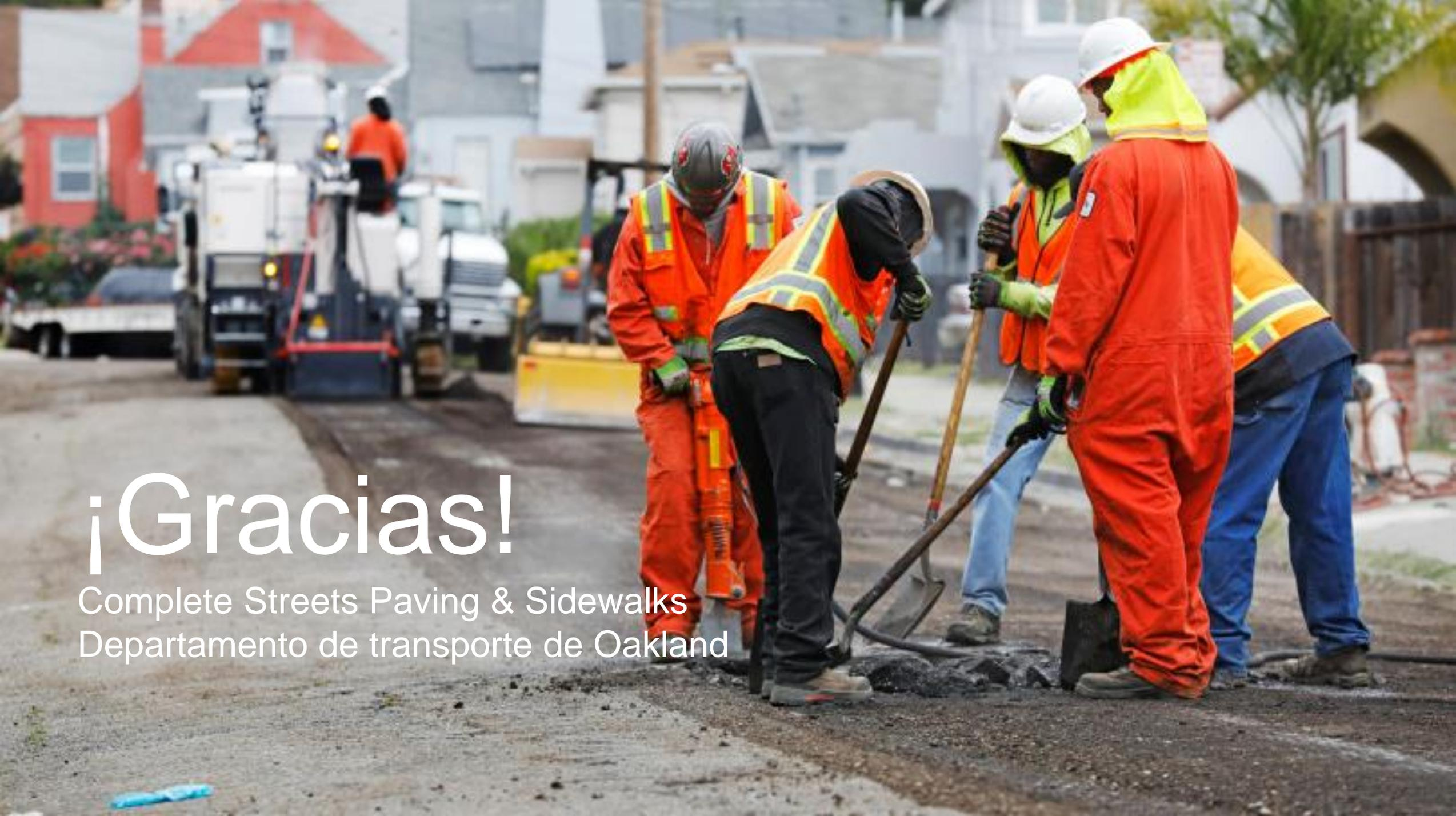
A group of construction workers in high-visibility orange and yellow safety gear are working on a street paving project. They are using tools like shovels and a tamper to compact the asphalt. In the background, a white paving machine is visible, along with residential buildings and a utility vehicle. The scene is set in an urban environment with a clear sky.
