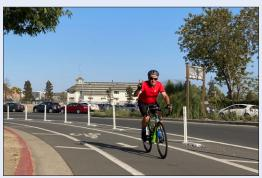
Vertical delineators separate bike lane from motor vehicles.
