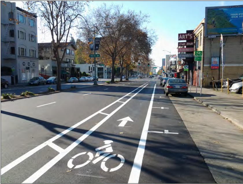
New striping on Broadway, 38th St to Broadway Ter, features buffer striping on both sides of the bike lane.
