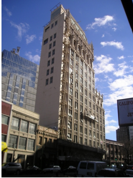
Figure 14 – view from 17 th Street and Telegraph
