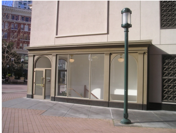
Figure 11 – Storefront at down stairwell, from Kahn's Alley
