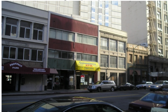
Figure 16 – Low use windows at 2 nd and 3 rd Floors
