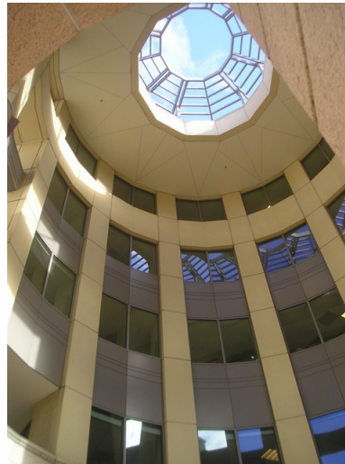
Figure 5 – View inside Rotunda
